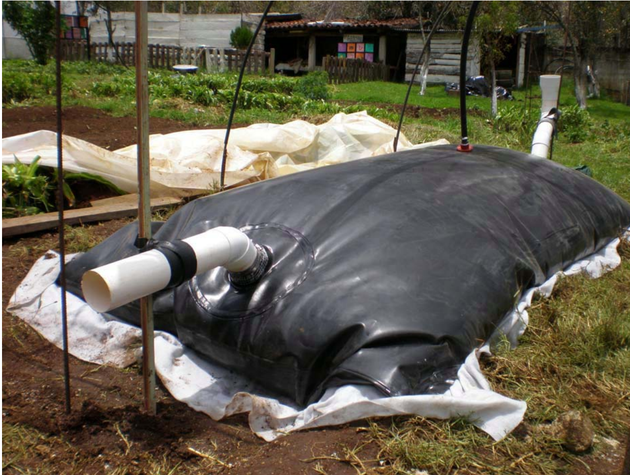
Figure 2. Plug flow biogas digester in Chiapas under construction
